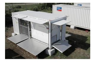
Today, solar energy covers 46% of St. Eustatius' total electricity need. Grid Forming SCS 2200 inverters allow to operate the island grid for 10.5 hours in Diesel Off-Mode operation with 100% Solar Power Fraction. In total a 5.9MWh Li-lon storage facility has been integrated for energy shifting and grid services. Thanks to the SMA Fuel Solution about 4,560 tons CO2 per year can be saved. The project has been designed, and implemented by the SMA Sunbelt Energy GmbH.
