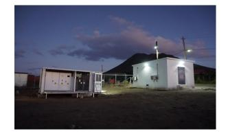
Today, solar energy covers 23% of St. Eustatius' total electricity need. To stabilize the grid, which is influenced by fast power fluctuation related to cloud movement, a Li-lon storage facility has been integrated to absorb the fluctuations, provide energy shifting and frequency stability functionality also at night. Thanks to the SMA Fuel Solution about 2,240 tons CO2 per year can be saved. The project has been designed, and implemented by the SMA Sunbelt Energy GmbH.
